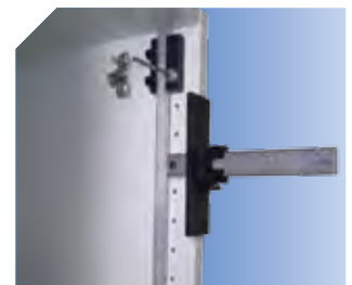
Drilling for placing invisible hinges.
