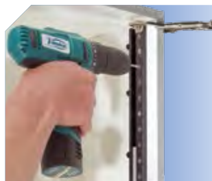
Drilling for placing shelves.
