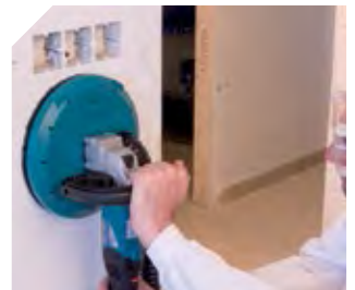
It allows to sand the walls even in difficult areas.
