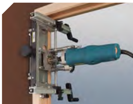
Making the upper recess on the frame.
