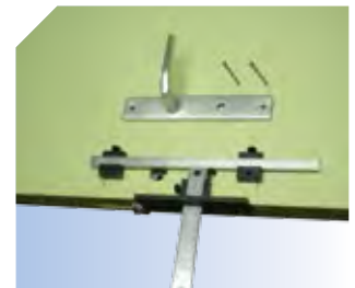
Drilling for door accessories.
