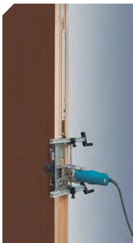
Making the second recess on the frame.
